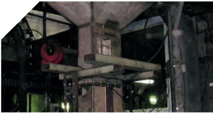
**MoistScan®** MA-600 installed on the wall of a hopper feeding a briquetting press at a briquetting factory. The material is a mixture of sand, sodium nitrate and char. Control of the moisture content of the briquettes is critical. If the mixture is too dry the briquettes don't form correctly. If the mixture is too wet the briquettes may split in the fluidised bed dryer or in transit.
